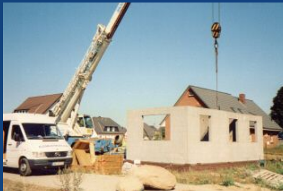
b) Precast systems based of anhydrite binder
